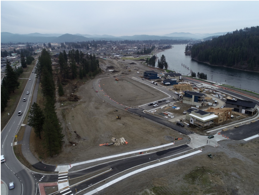
SITE PHOTO 8 - Drone Photo Looking at Areas 1, 2, 8, 10, and 12, and Seltice Way:
